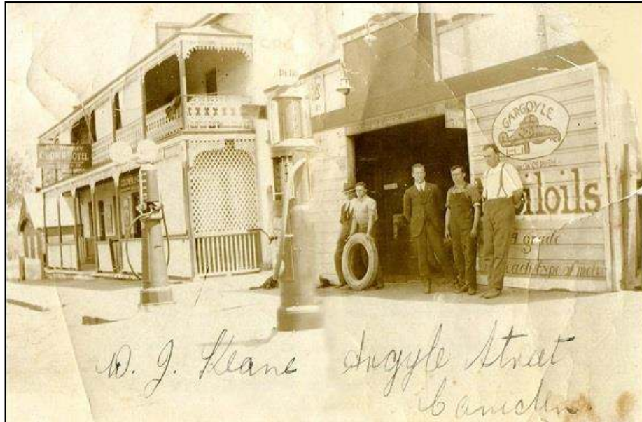
The garage at 177-185 Argyle Street that was purchased by John Souter in the 1940s. Here the garage is owned by DJ Keane in the 1920s with the Crown Hotel next door and the Show Hall Pavilion in the distance without its current frontage. The forces of motoring and Interwar modernism combine with a frontage on the Hume Highway. (Camden Images)
